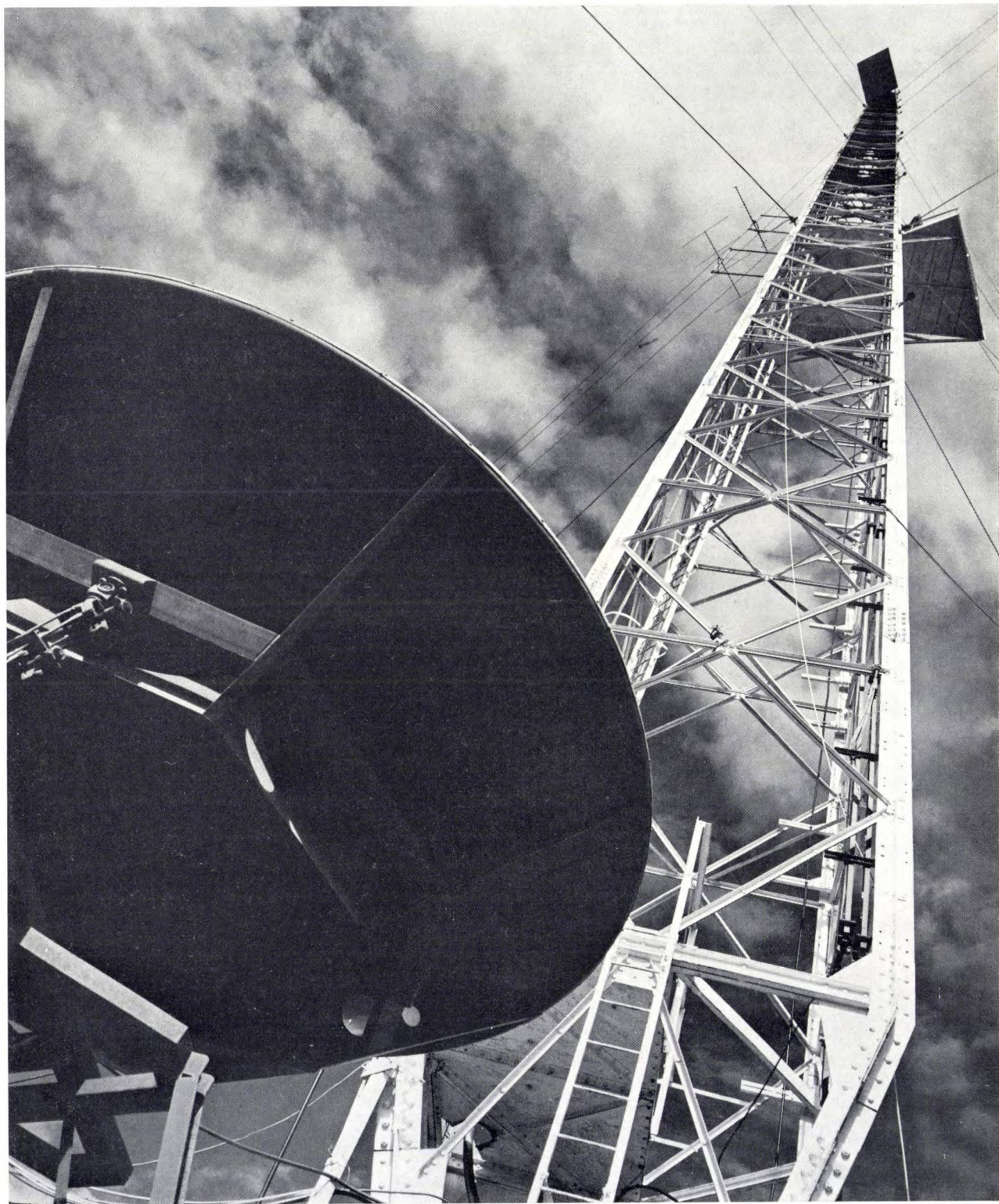
Fig. 3. Between 1950 and 1957 a considerable amount of work on "line-of-sight" microwave beam links was done at LEP in cooperation with TRT. The link between Bordeaux and the Pic du Midi (in the Pyrenees), established in 1957 using a multi-reflex klystron, at the time represented a world record: a high-definition television broadcast was transmitted directly over a distance of 213 km. The photograph shows the aerial system of the Bordeaux transmitter, with a parabolic antenna at ground level and a rectangular passive reflector at the top of the mast.
